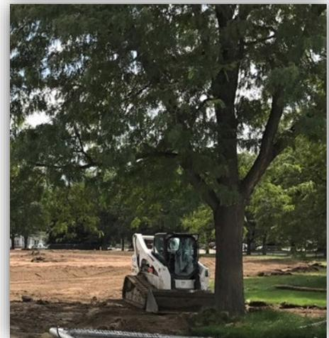
**Figure 3.** Heavy equipment traffic compacts soils.
