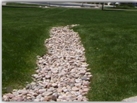
Figure 1. A French drain is a ditch-like trench filled with rock. Water must flow downhill to an outlet.
