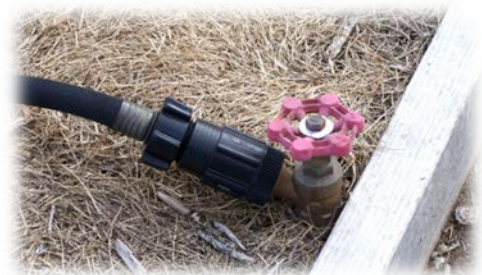
Figure 11. Tap, pressure regulator (with hose connections) and half-inch drip hose in raised bed garden.
