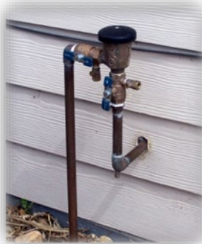
Figure 2. Required by local building codes, backflow prevention devices are typically located where the line comes outside from the house.
