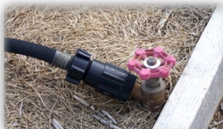
Figure 11. Tap, pressure regulator, hose connection, and half-inch drip hose in a raised bed garden.
