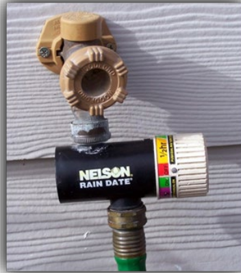
Figure 12. Single-zone controllers connect to the hose line. Left: This style is manually turned on and automatically turns off after a set number of minutes. Right: This battery powered controller turns water on and off at the day and time intervals set by the gardener.
