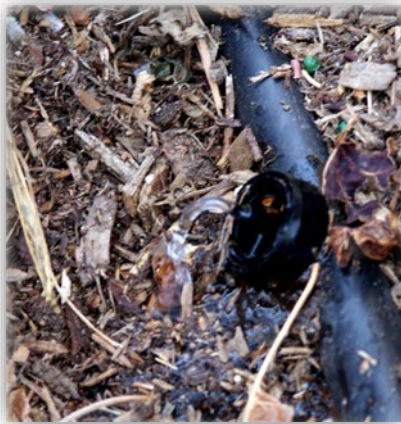
Figure 10. Drip emitter on ½" poly tubing.
