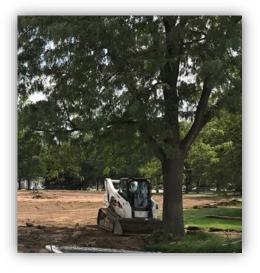
Figure 3. Heavy equipment traffic compacts soils.
