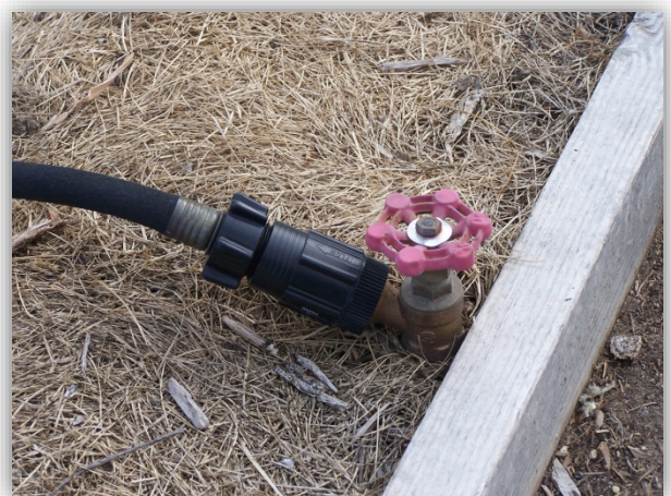
Figure 4. With irrigation pipe, it is easy to plumb a tap at each raised bed box. Here a pressure regulator with hose-end fittings reduces pressure to 25 psi. It is connected to a ½-inch soaker hose.
