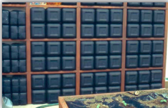
Figure 2. Milk jug water storage wall in a passive solar hobby greenhouse. Disposable milk jugs on left and returnable milk jugs on right are spray painted flat black. In this well-built structure, nighttime temperatures dropped to 39°F with no supplemental heat when outside temperatures dropped to -17°F.
