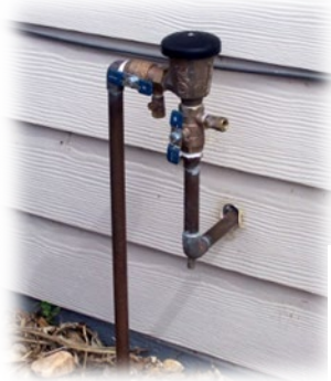
Figure 2. Required by local building codes, backflow prevention devices are typically located where the line comes outside from the house.
