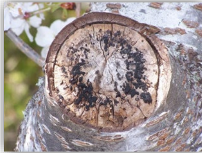
Figure 15. The black material in the pruning cut is decay fungus. Notice the cracking; it also raises flags of structural integrity.
